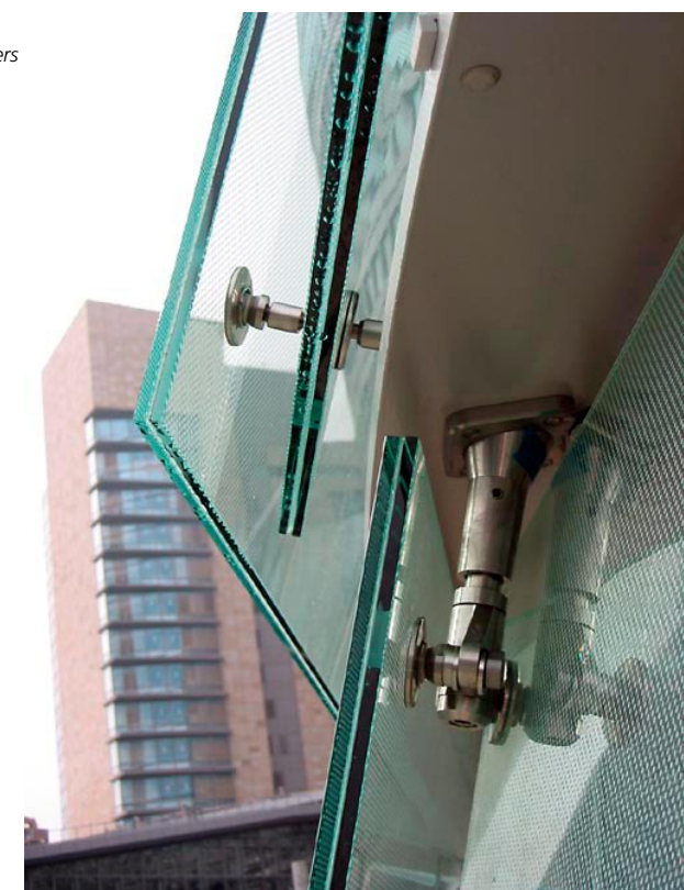
Figure 8 Glass holder details (Scale 1:10)
