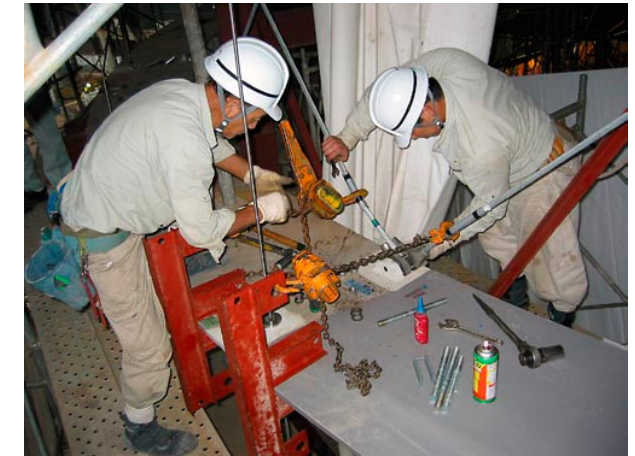
Figure 15 Cable tensioning
