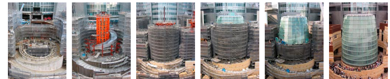
Figure 17 Erection sequence
